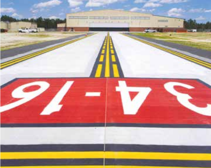
Unmanned Aircraft Vehicle (UAV) Hangar and Runway MQ-1C Gray Eagle, Camp Mackall, North Carolina
