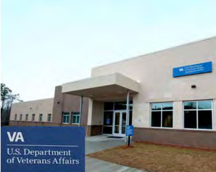
VA Austell Primary Care Clinic Austell, GA
