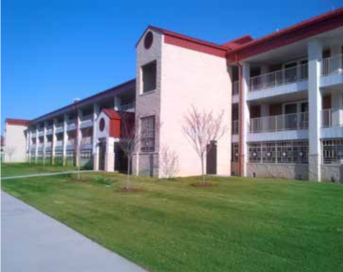
TBUP Barracks Renovation FY12, FY13, FY14 6 Buildings, 61,000 SF/building Fort Gordon, Georgia
