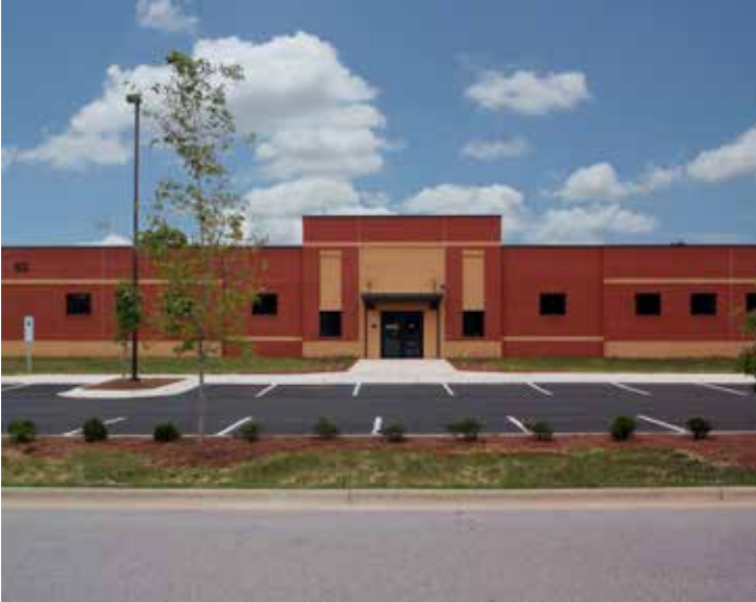
Linden Oaks MEDCOM Womack Facility Cameron/Fayetteville, North Carolina
